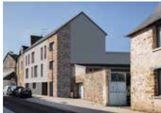
La Mériaïs, Vitré (35) PRISM ARCHITECT
